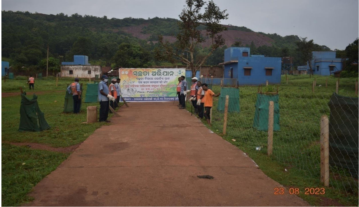
Photograph of Concrete Road after cleaning
